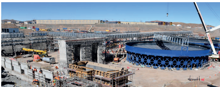
Teck Resources' QB2 project comprises a 143,000 t/d copper concentrator, a high-capacity desalination plant and a 165 km water supply pipeline (credit: Teck Resources)
