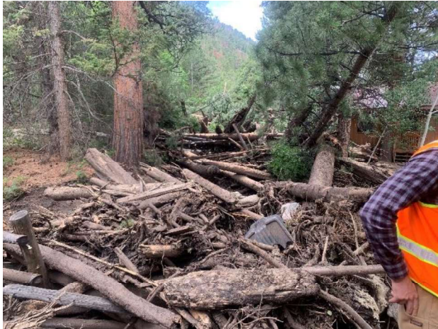
Figure 6. Debris dam of the drainage channel at the site.
