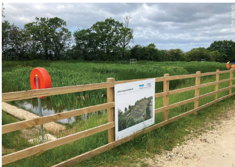
Above and below: Clifton Integrated Constructed Wetlands is Yorkshire’s first nature-based wastewater-treatment system
